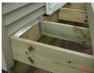
**Flashing:** Check to make sure it is sound and firmly in place
