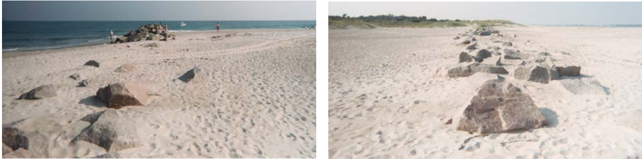
Figure 42: Existing rock groin at east end of Fort Macon State Park (August 2005).
