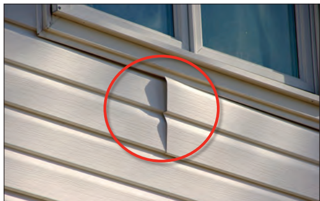
Figure 6. Proper detailing around windows and other obstacles is important. Use utility trim, punch snap-locks into siding, and do not overlap directly beneath a window.
