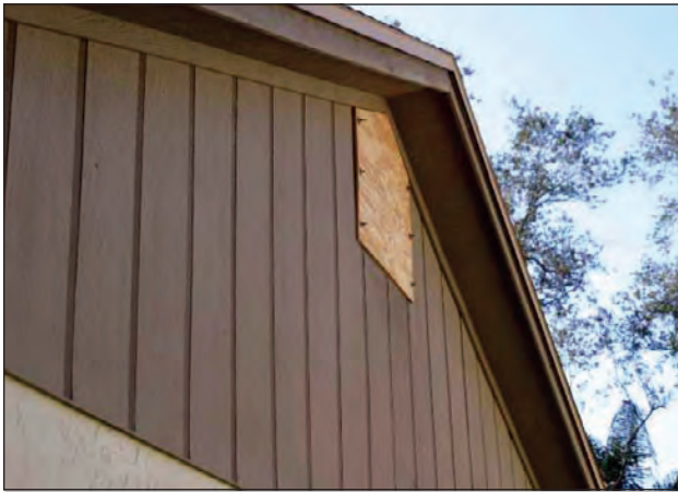
Figure 10. Shuttered gable end vent.
