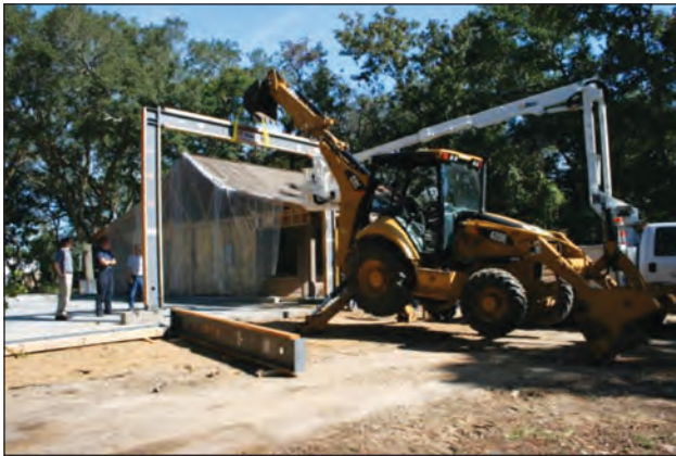
Figure 4. Installation of a prefabricated ordinary moment frame.
