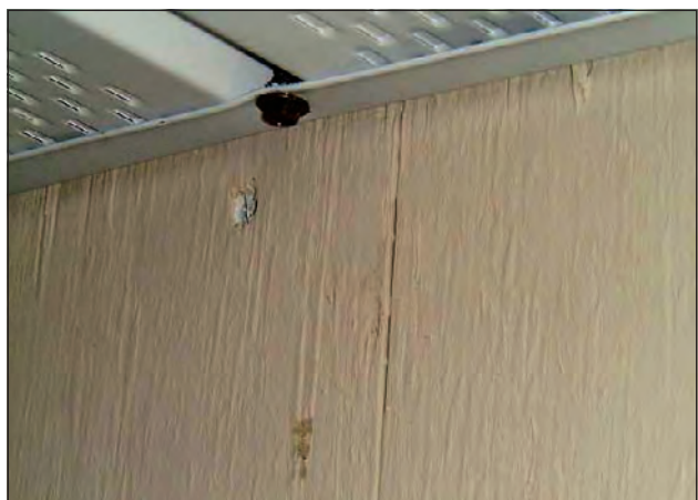
Figure 5. Screws through wall channel.
