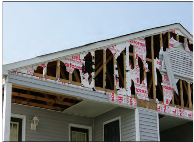
Figure 7. The vinyl siding at this gable was installed over plastic foam insulation. Without wood sheathing, the wind pressures on the vinyl are increased. Also, if the siding blows away, the foam insulation is very vulnerable to blow-off. With loss of the foam insulation, wind-driven rain can freely enter the attic, saturate the ceiling insulation, and cause collapse of the ceiling.
