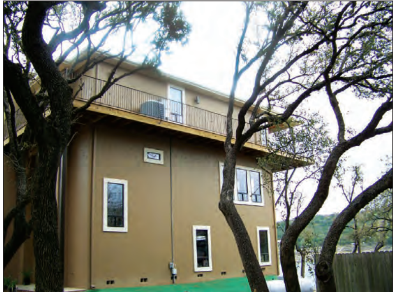
Figure 7. Example of a two-story enclosure below the BFE. This type of enclosure presents special construction and flood insurance issues. Contractors should proceed with caution when an owner requests such an enclosure.
