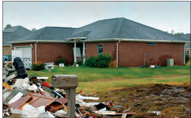
Figure 1. Bridge City, Texas, homes were flooded during Hurricane Ike, even though they were constructed outside the SFHA and in Zone B. The flood level was approximately 4' above the closest BFE.
