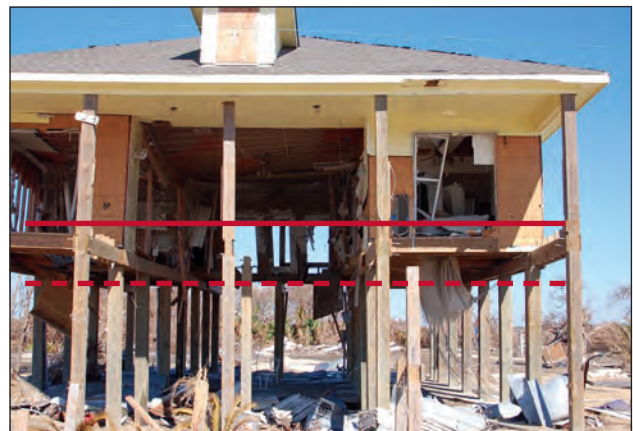
Figure 2. Bolivar Peninsula, Texas, V Zone house constructed with the lowest floor (bottom of floor beam) at the BFE (dashed line). The estimated wave crest level during Hurricane Ike (solid line) was 3' to 4' above the BFE at this location.
