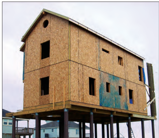
Figure 2. Construction of a Structural Insulated Panel house.
