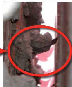
Figure 7. Misalignment of the tie reduces the embedment and promotes veneer failure.
