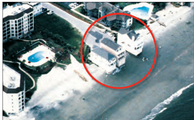
Figure 1. Well-built but poorly sited building.
