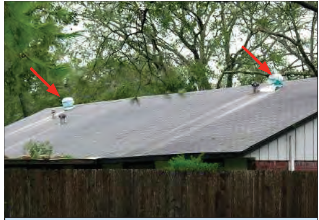
Figure 14. Plastic wrapped turbines.
