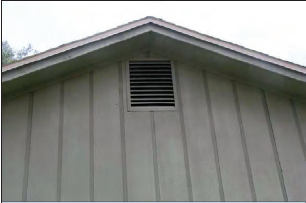
Figure 9. Gable end vent.
