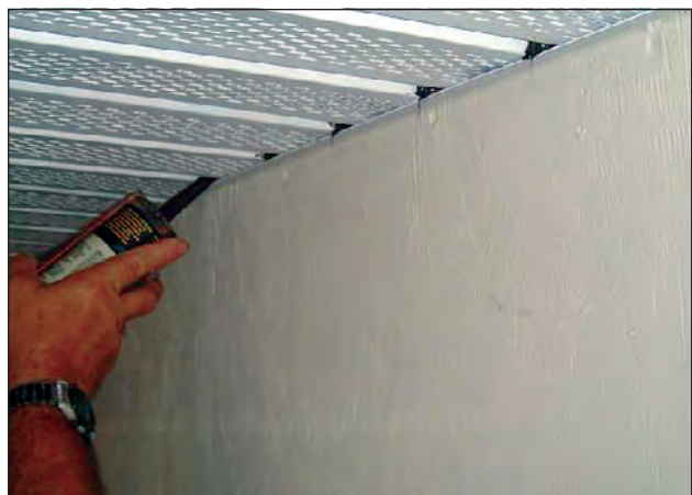
Figure 4. Applying dabs of sealant.
