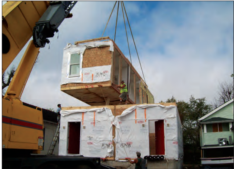
Figure 1. Construction of a modular home.
