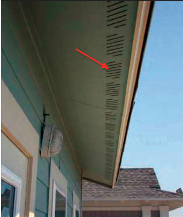
Figure 6. Fiber cement soffit with ventilation slots (red arrow).
