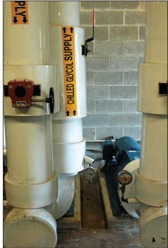
Figure 5-4. Chilled water pump, Georgetown, Delaware.
