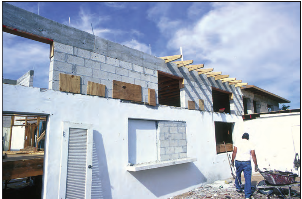
Figure 67 The extended first-story walls.
